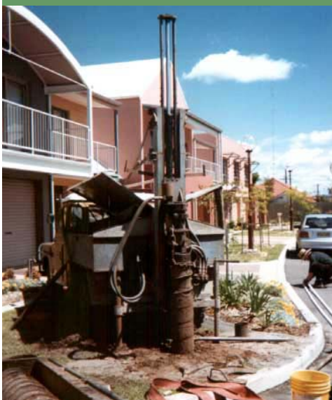
Photo: Installing a groundwater bore (Sourced from HCCREMS)
