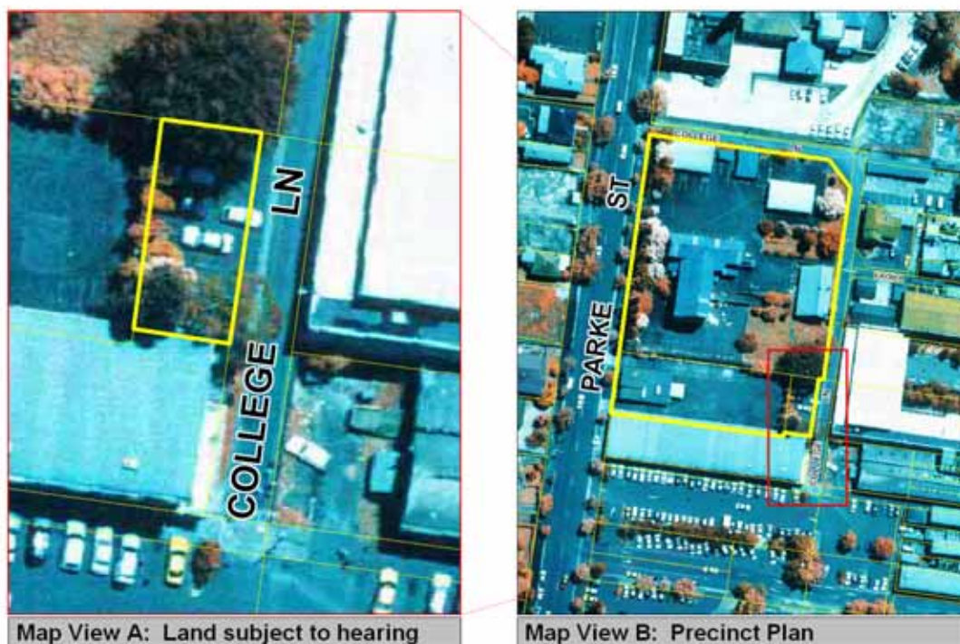
Figure 2: Aerial photographs of subject land (Map View A) and in the context of the larger Katoomba Cultural Precinct Setting (Map View B). 2
