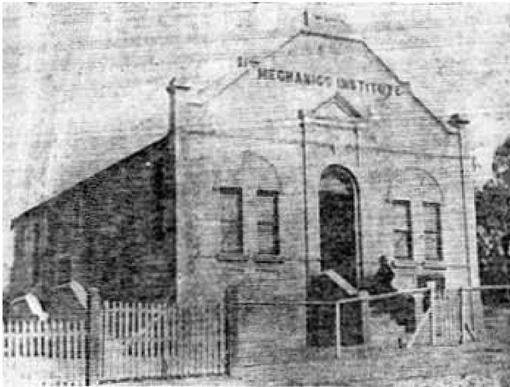
FIGURE 2: Original façade c.1905 (BM Historical Society, reproduced in NBRIS, p. 12)
