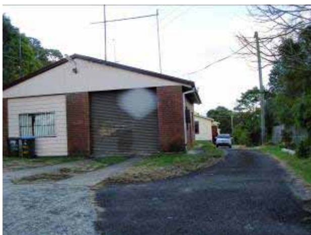
FIGURE 7: View north alongside RFS building
