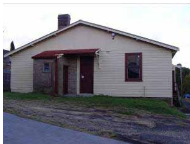
FIGURE 8: Rear of Mechanics Institute, 1930's additions
