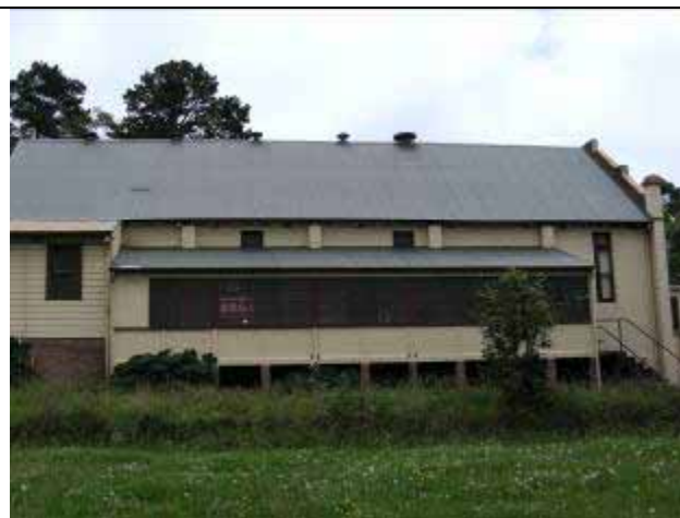
FIGURE 6: Eastern façade – front portion - verandah
