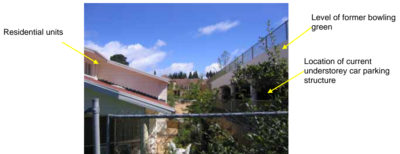
East-west view showing bowling green understorey car parking and residential units. March 2005.
